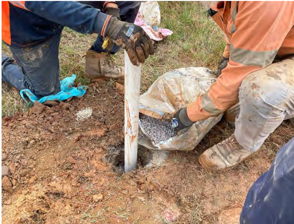
Photo 11 - Bentonite pellets used as an annular seal & backfill for piezometers (BH09)
