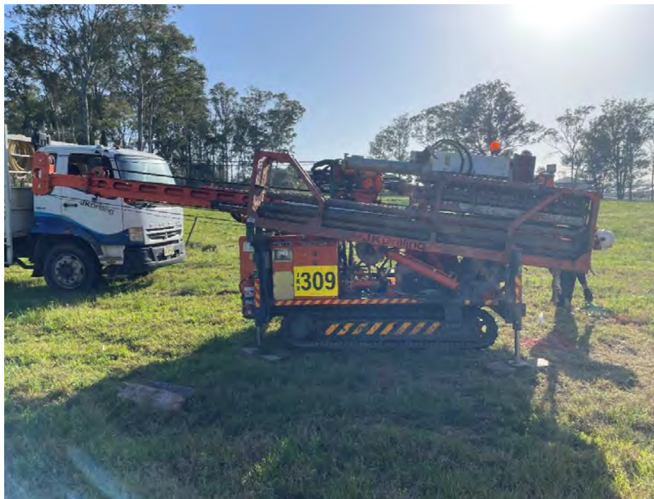
Photo 6 - 6-tonne track mounted drill rig used for BH07 & BH08 (photo taken at BH08)
