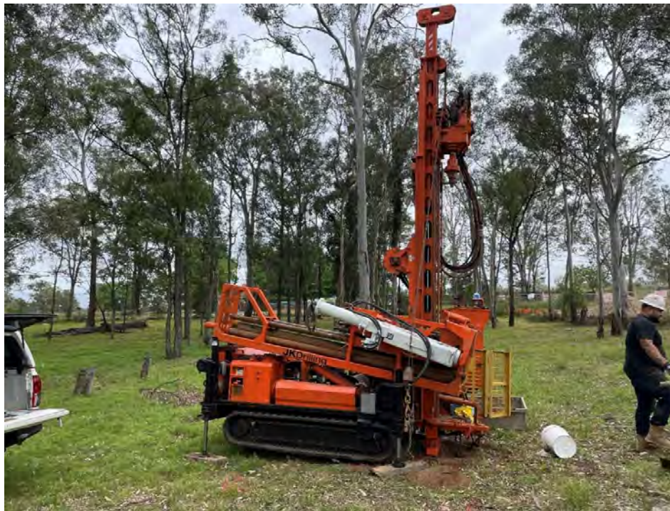
Photo 5 - 6-tonne track mounted drill rig used for BH05, BH06 & BH09 (photo taken at BH06)
